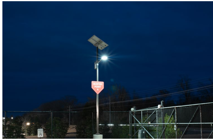
VIEW. Inc Olive Branch, MS Packing Lot Lighting Project
